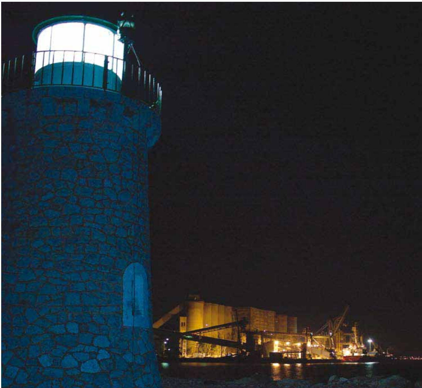
Patras Plant, Achaia, Greece
