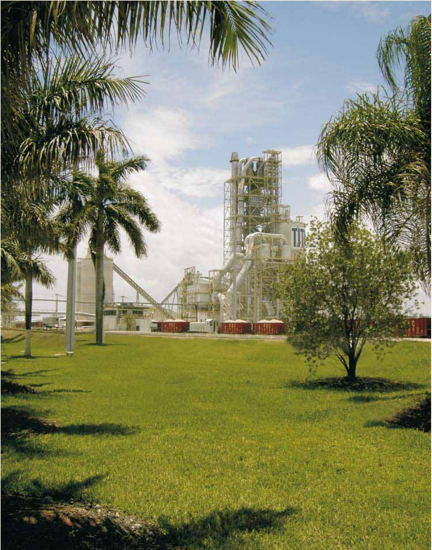
Pennsuco Plant, Florida, USA
