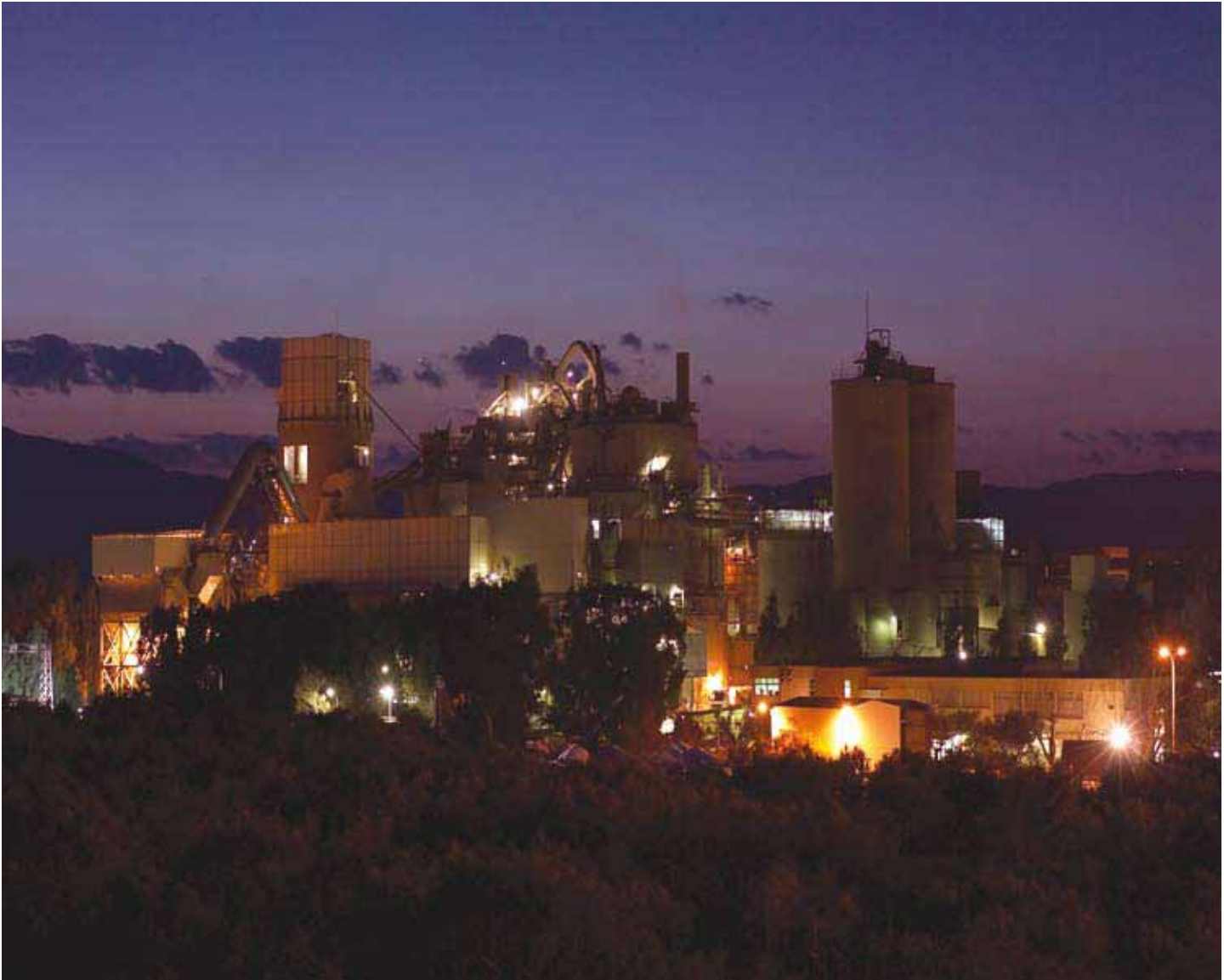
Patras Plant, Achaia, Greece
