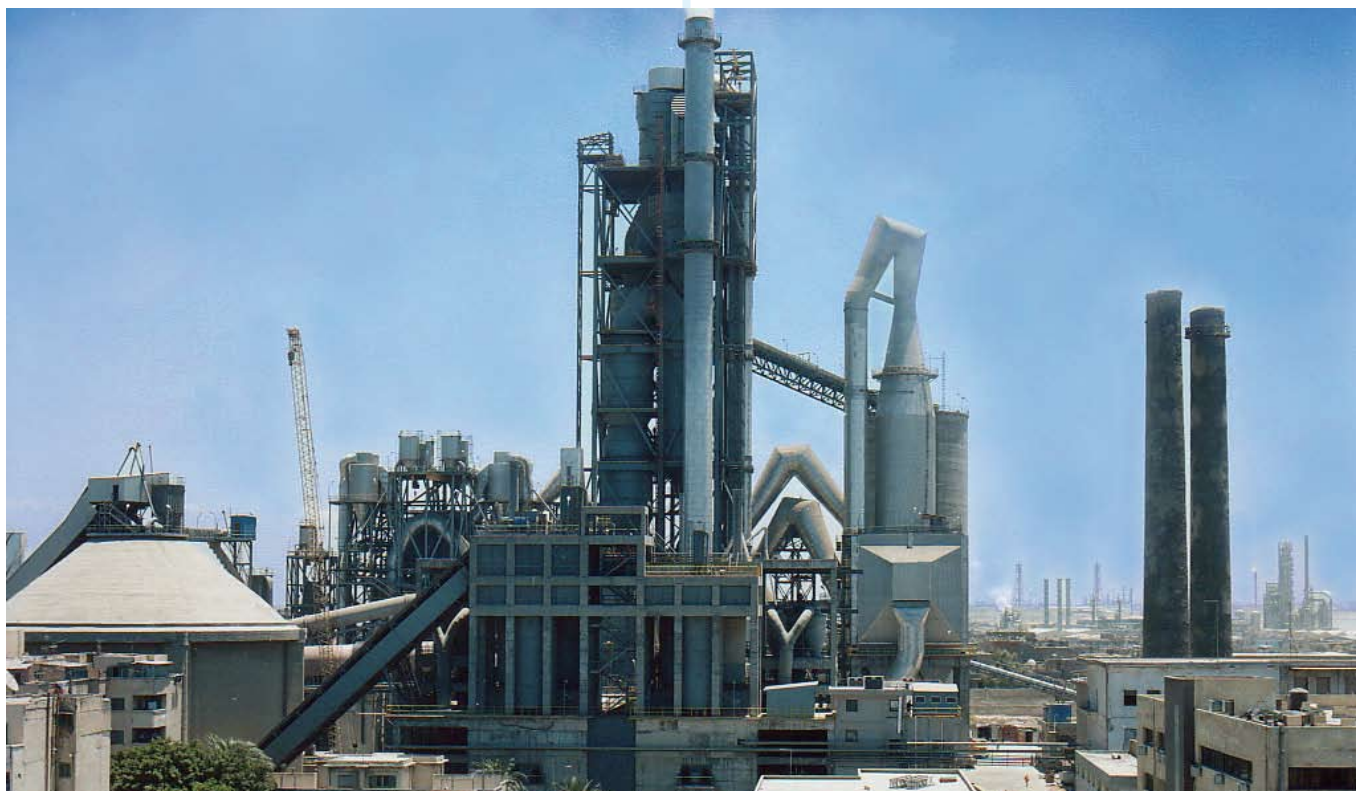
Alexandria plant, Egypt
