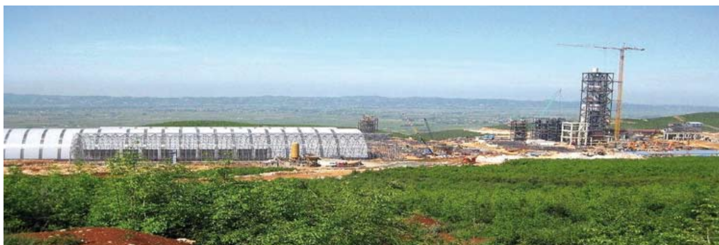
Greenfield cement plant under construction in Boka e Kuqe, Albania
