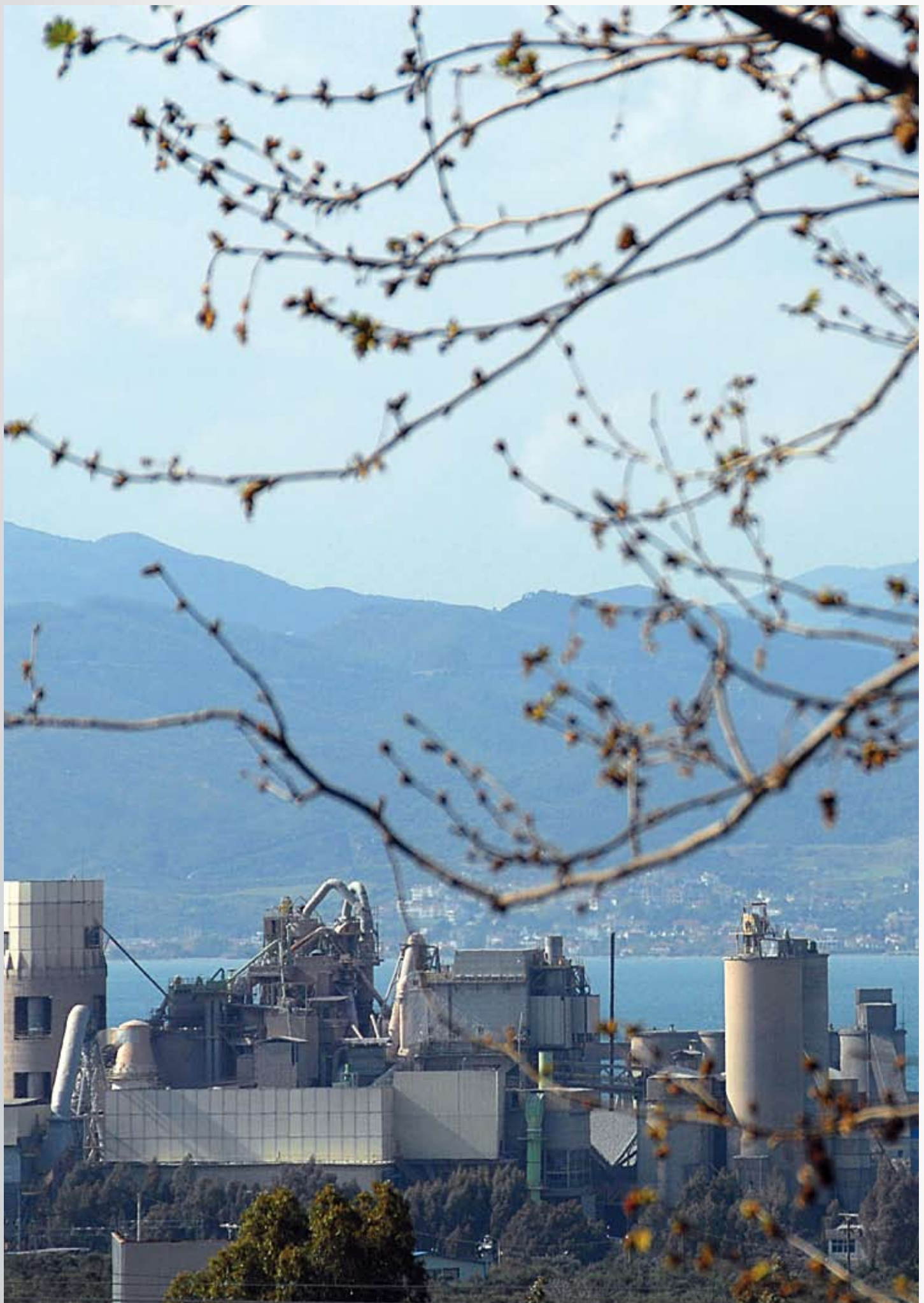
Drepano plant, Patra, Greece
