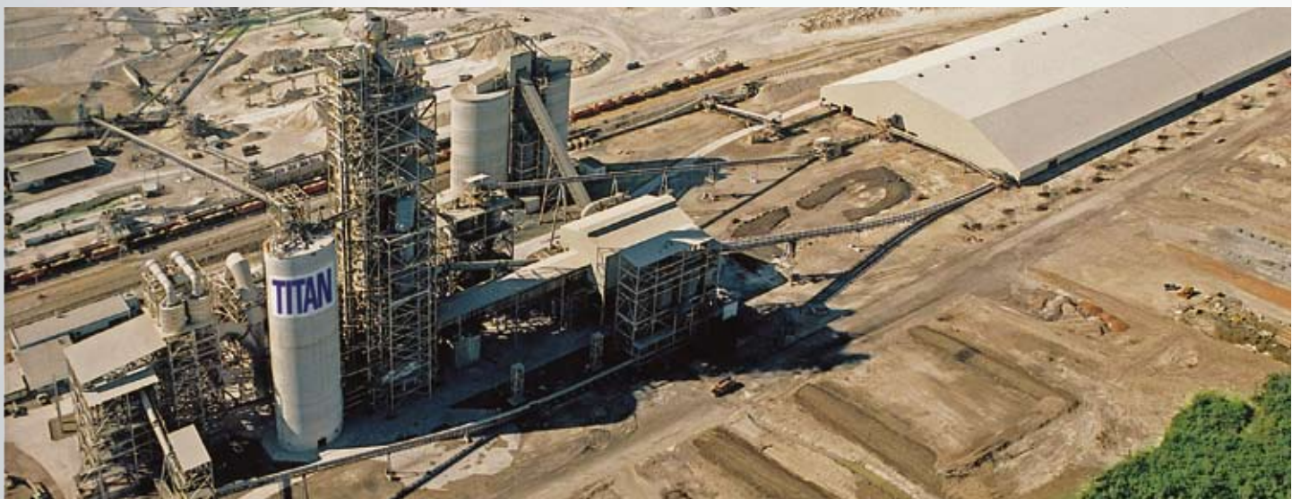
Pensuoco plant, Florida, USA
