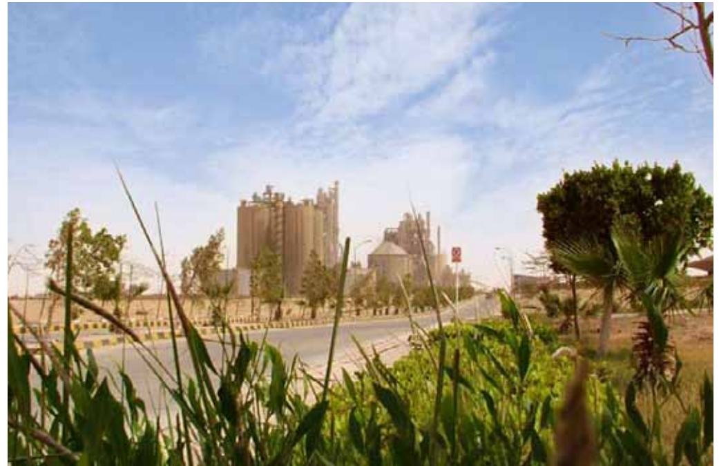
Beni Suef cement plant, Egypt
