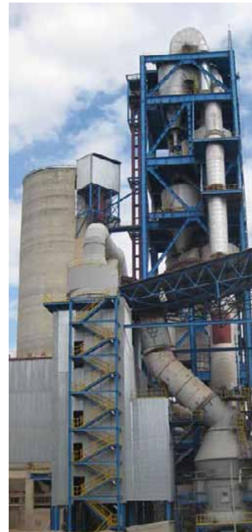
Adocim cement plant, Turkey
