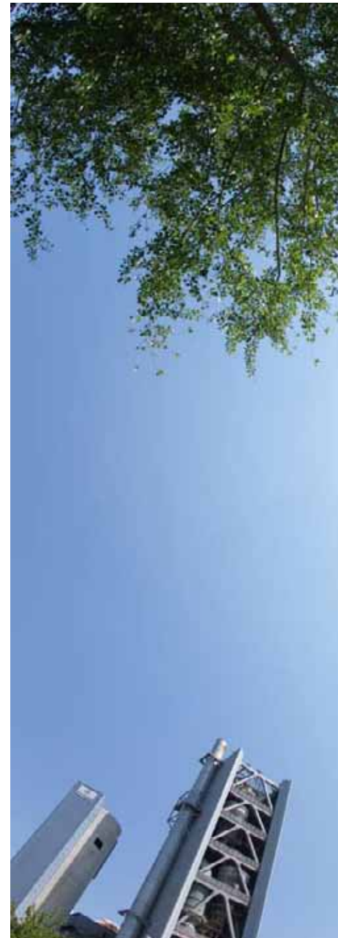
Thessaloniki cement plant, Greece
