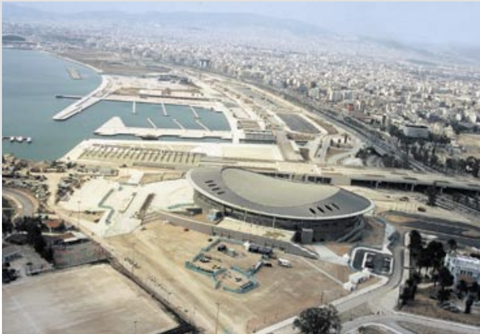
TAE KWON DO Olympic premises, Athens - Greece
