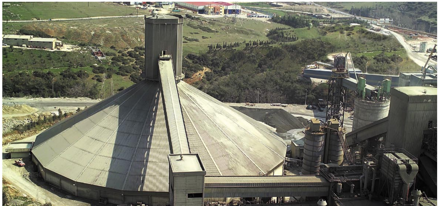
Clinker storage hall, Thessaloniki plant, Greece
