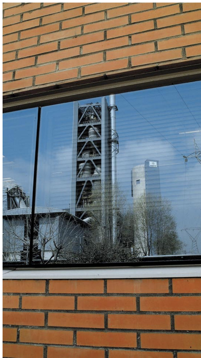
The new production line at Thessaloniki plant, Greece
