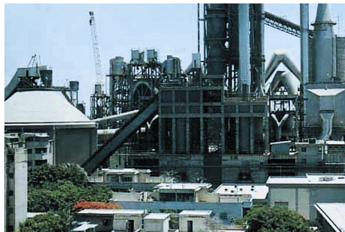
Alexandria plant, Egypt
