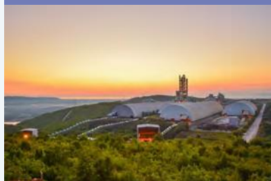
Antea cement plant, Albania
