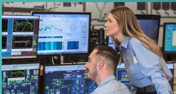
Control room, Kamari plant, Greece
