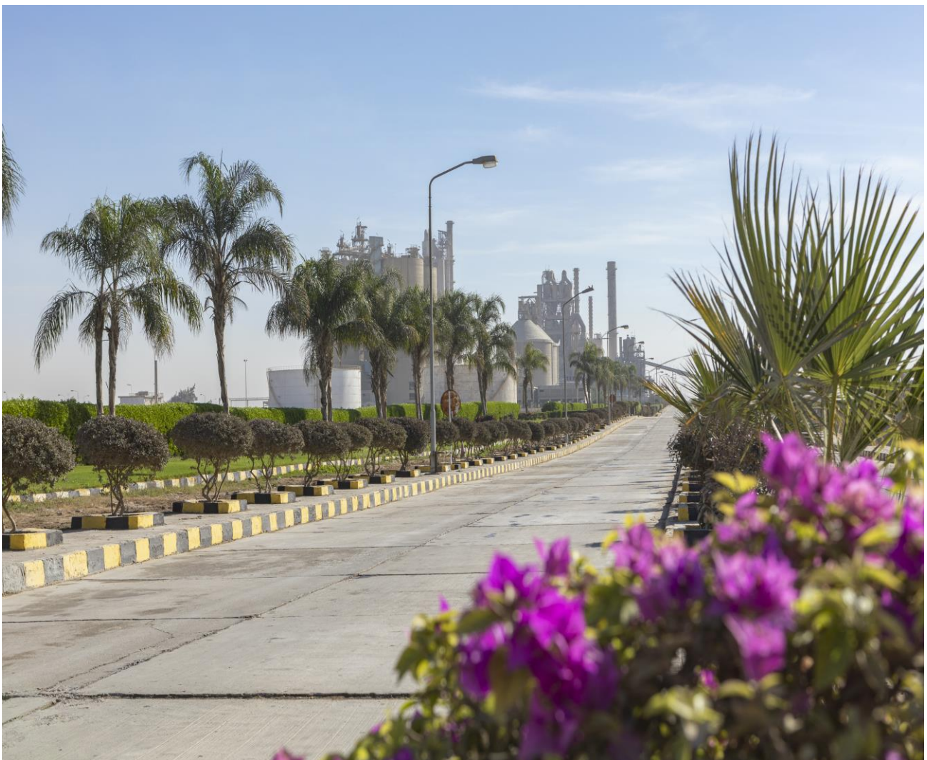
Beni Suef cement plant, Egypt
