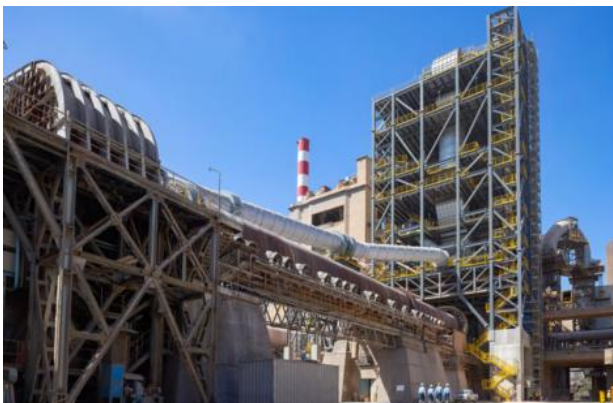
State-of-the-art pre-caliner technology at Kamari plant, Greece
