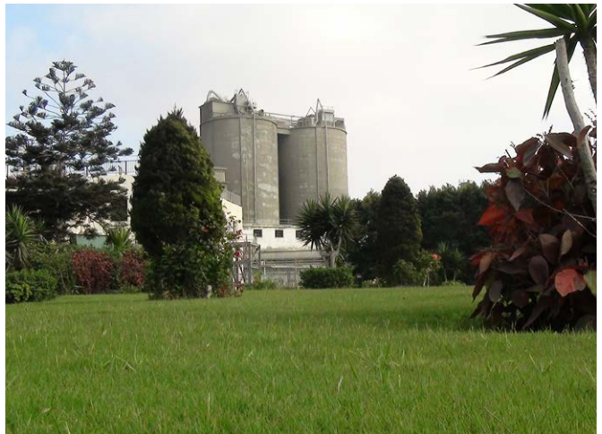
Alexandria cement plant, Egypt
